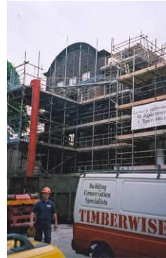
1761 Building during refurbishment works
