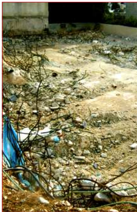
Before one day in July 2008 a four-storey house stood here. Its demolition made 70 people homeless.
